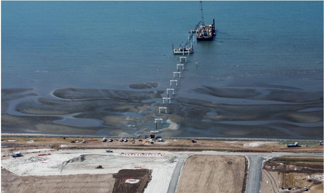
Installation of new Runway Lighting
