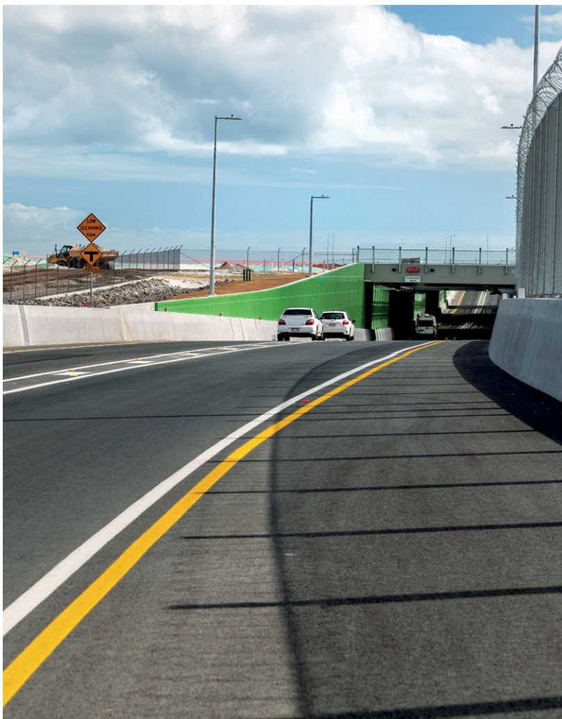
Dryandra Road Underpass
