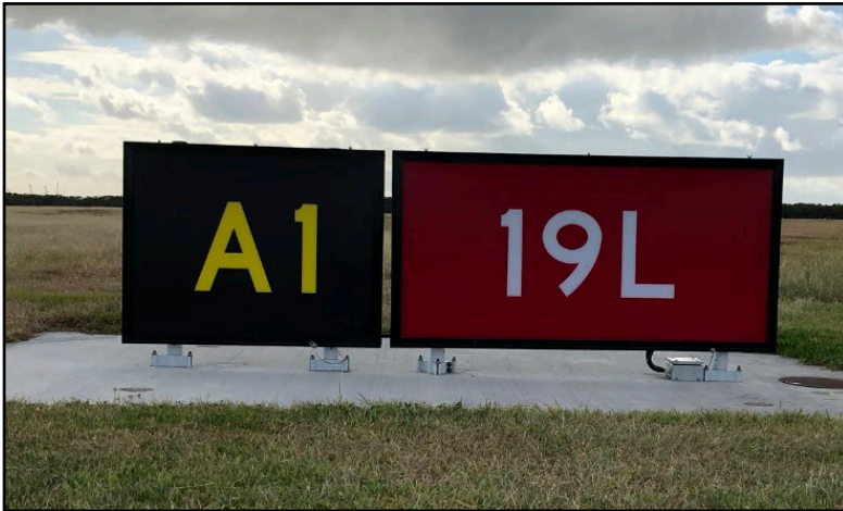
Figure 63 Runway Designation Sign
