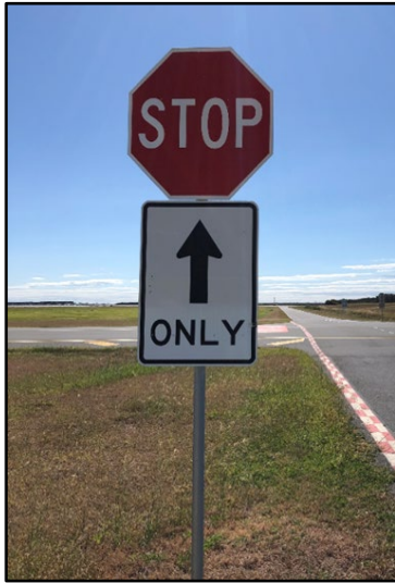
Figure 17 Taxiway Crossing Stop Sign Example
