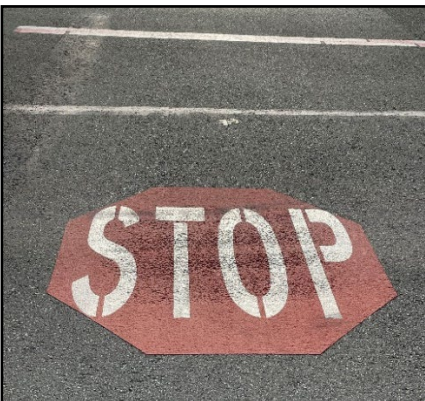
Figure 14 Painted Stop Signs
