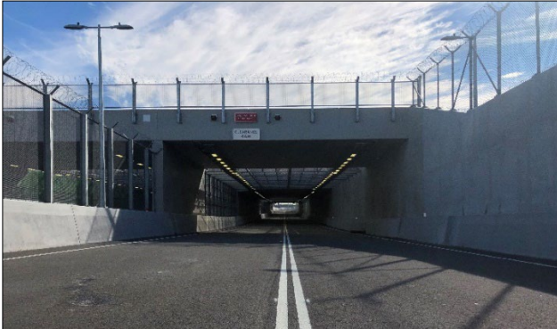
Figure 1 Dryandra Road Underpass Height Restriction
