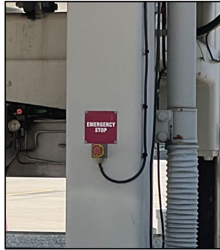
Figure 25 Aerobridge Emergency Stop Button
