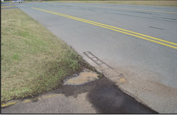
Figure 31 Example of leaving paved areas resulting in mud, grass and gravel on taxiway
