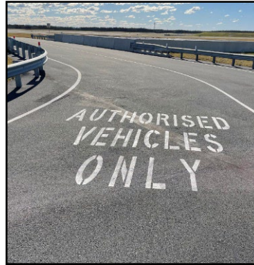
Figure 30 Authorised Vehicles Pavement Marking
