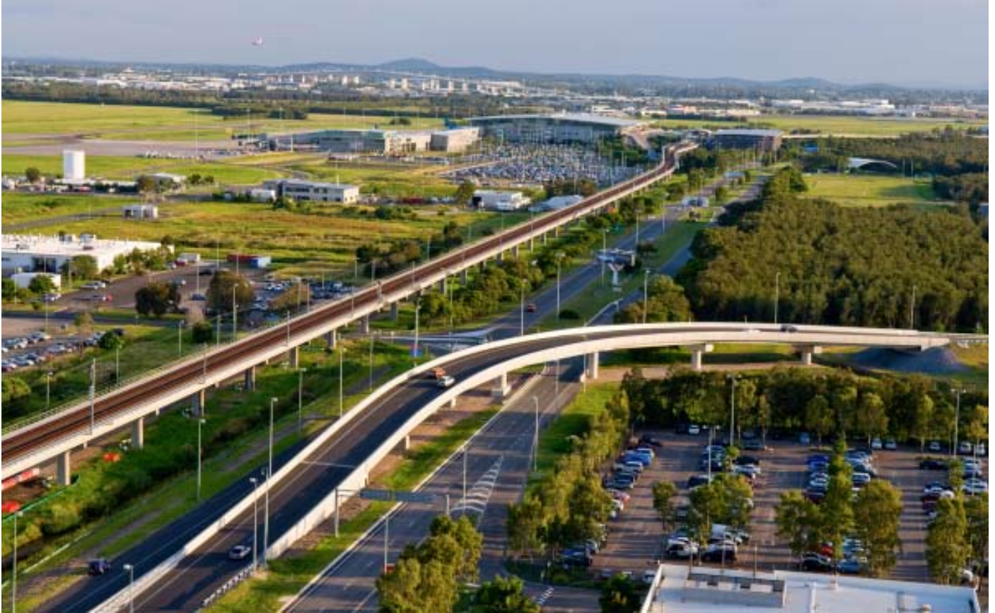
Brisbane Airport as seen from the Airservices Australia Control Tower
