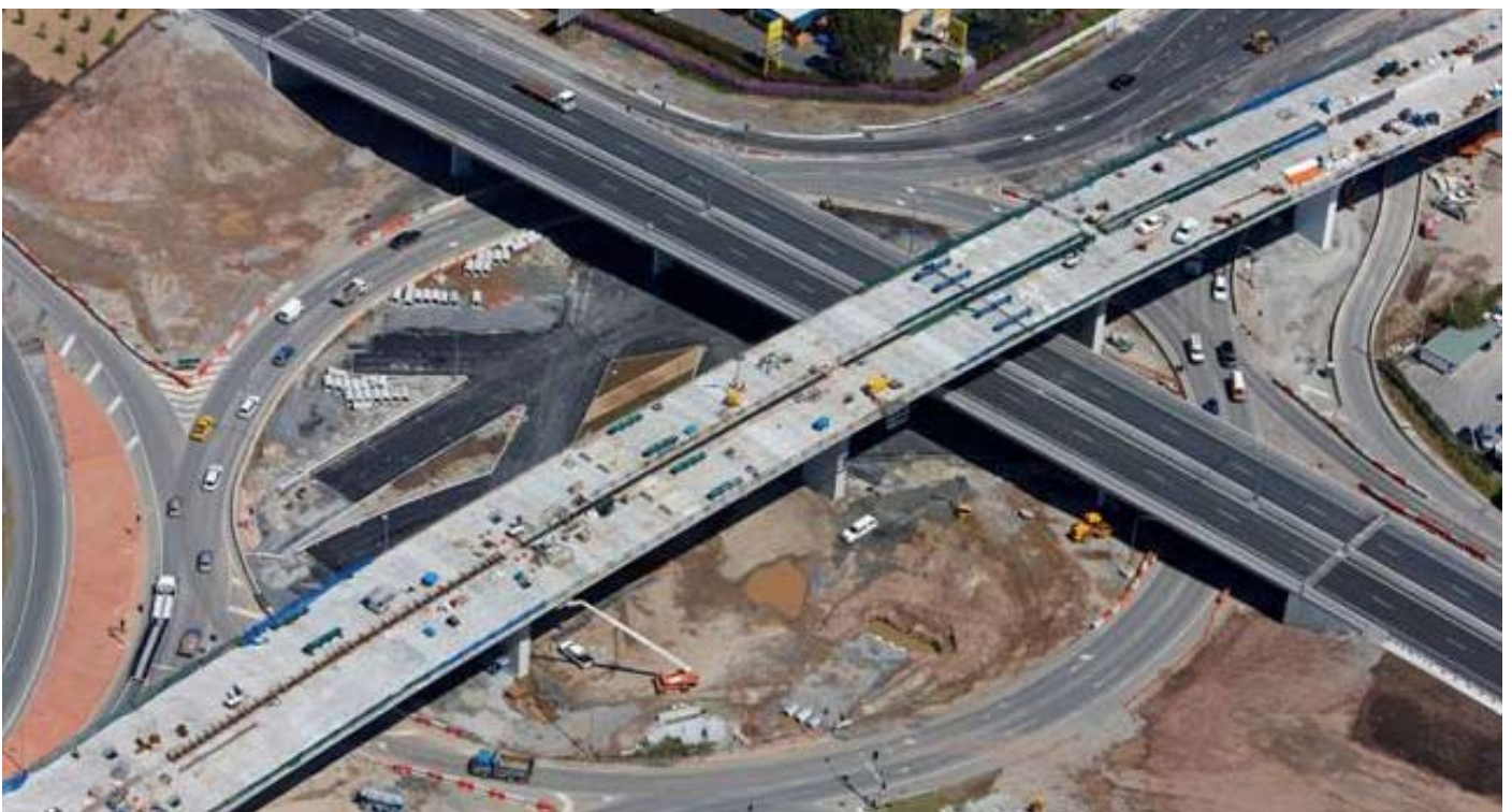
The Airport Roundabout Upgrade project makes progress
