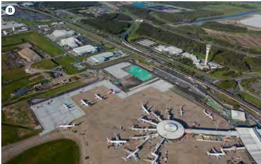
A. Artist's impression of the Brisbane Airport Hotels and Conference Centre development B. Southern apron expansion at the Domestic Terminal
